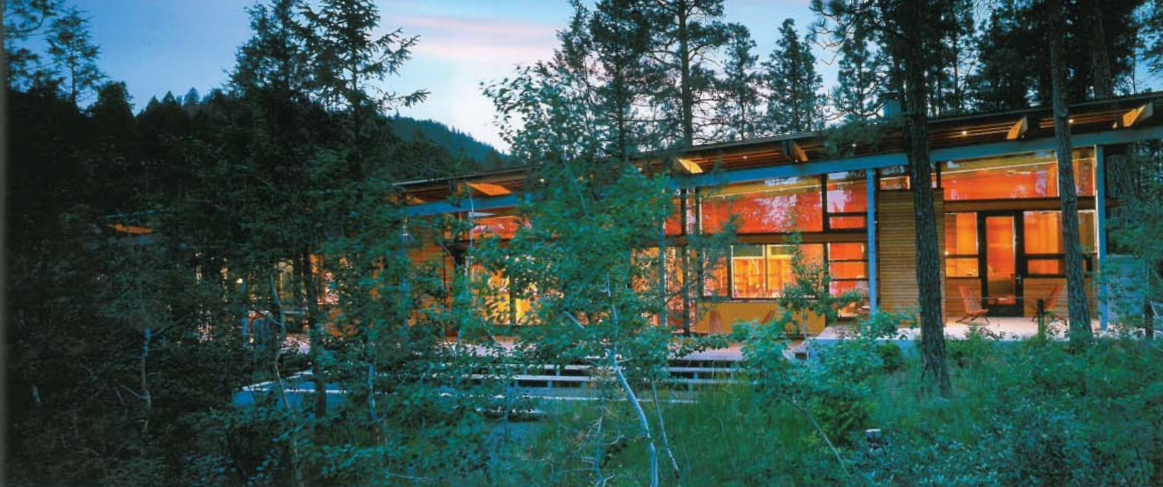
暮色中，透過湖畔的松樹、白楊和柳樹林能隱約看到坡形屋頂下發光的住宅空間。階梯和露臺上青草點綴的沙礫小徑在住宅和場地間形成過渡。At dusk, the house is an illuminated space under the sloped roof seen from the lake through a forest scrim of pine, aspen, and willow. Stairs and decks make the transition between the house and the site with grass gravel paths. (Photo by: Nic Lehoux)
