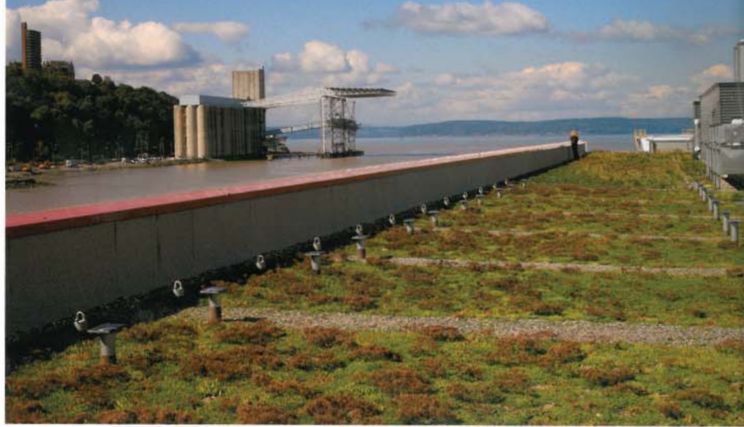
大樓綠色屋頂景觀一角 One of the building's green roofs (Photo by: Swift Company)
