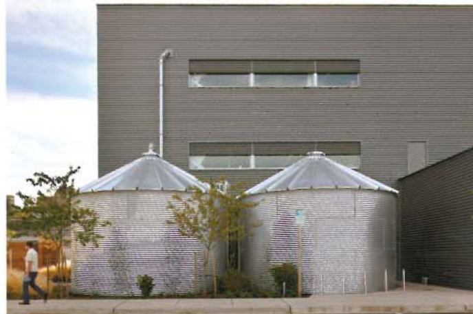
貯水槽主要收集屋頂徑流雨水及過剩的實驗蒸餾水，可提供抽水馬桶用水和場地灌溉用水 Cisterns for reclaimed roof and lab water for reuse for irrigation and toilet flushing (Photo by: ben benschneider)
